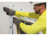
ance requirements that allow it to be left exposed up to 180 days, the self-adhering flashing features a treated release film on its adhesive side. Joining the company's extensive waterproofing solutions, the flashing comes in 4-, 6- and 9-inch rolls that fit a range of projects. **Circle 180 on inquiry card**
